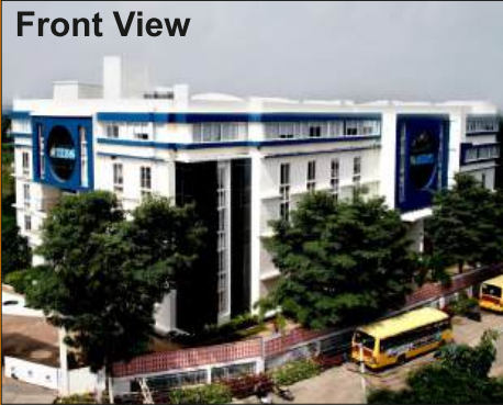
Airport Campus Bengaluru
